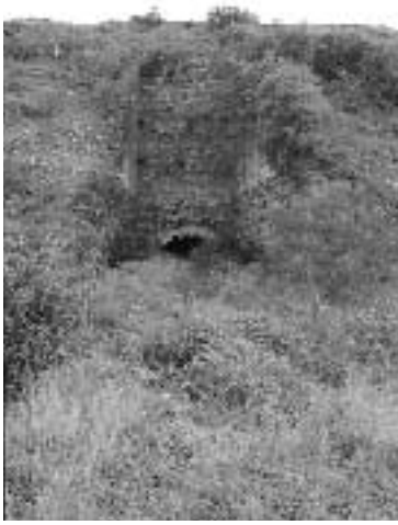
Fig. 7. Shaft kiln at Limeburner's Point, Geelong, showing front retaining wall, remnant wing walls and top of vault (Heritage Victoria)
